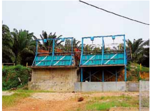
FFB Ramp using chain block door system
