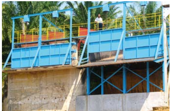
FFB ramps using chain block door system
